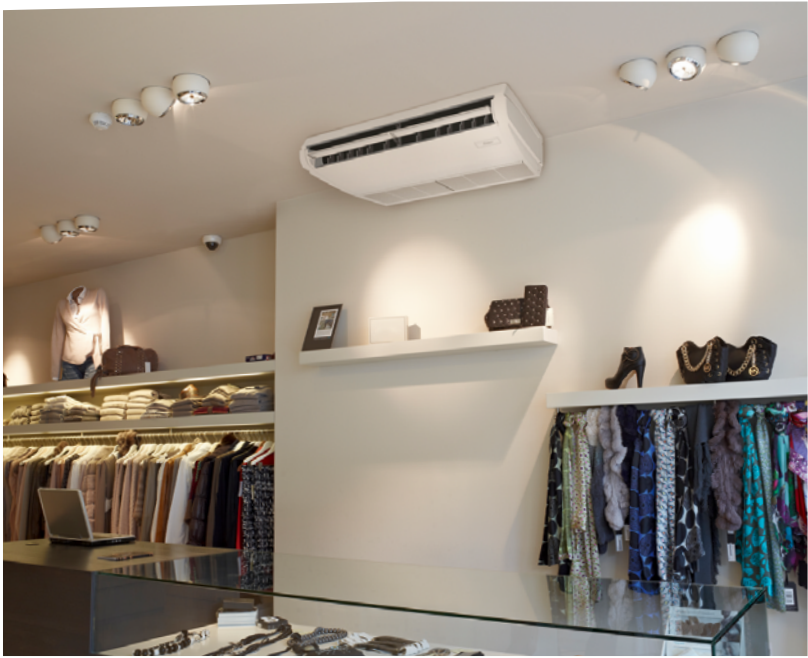
Ceiling suspended unit
